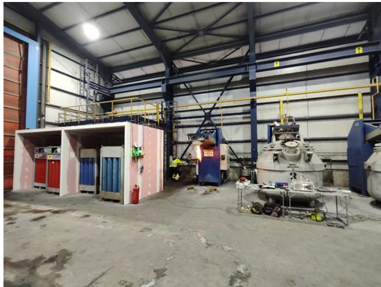
Figure 4: Test flame without ladle for confirmation
