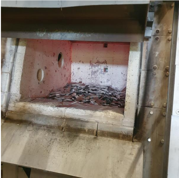
Figure 22: Scrap charged into melting furnace for dross test.
