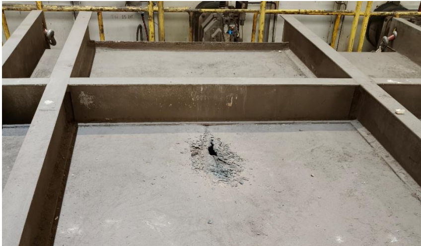
Figure 17 Lid broken by the loose refractory
