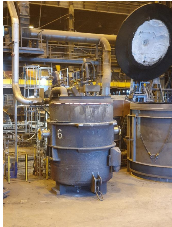
Figure 146. The ladle heater during the hydrogen test at around 3 hours after start-up.
