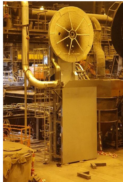
Figure 130. Photo of the ladle heater shortly after installation on site.
