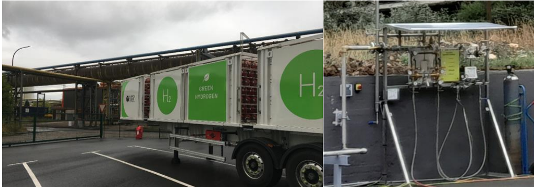
Figure 5. Hydrogen supply and decompression station at AMI.
