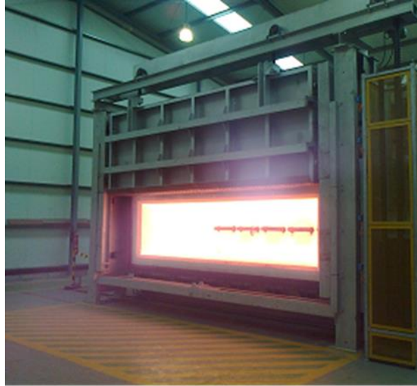
Figure 9. Long-term testing AMI direct heated combustion chamber.
