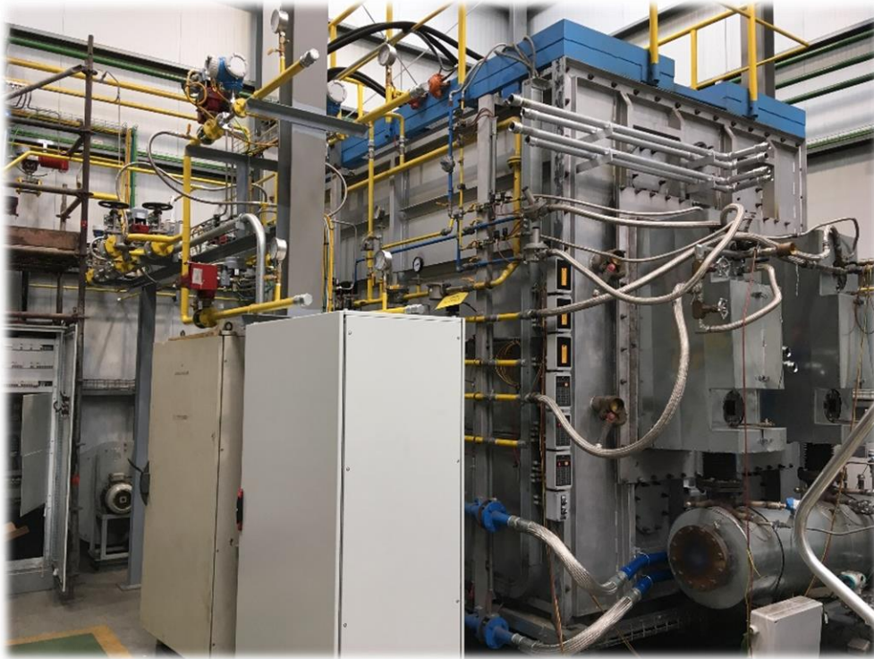
Figure 38. AMI pilot scale combustion chamber at Gijon site.
